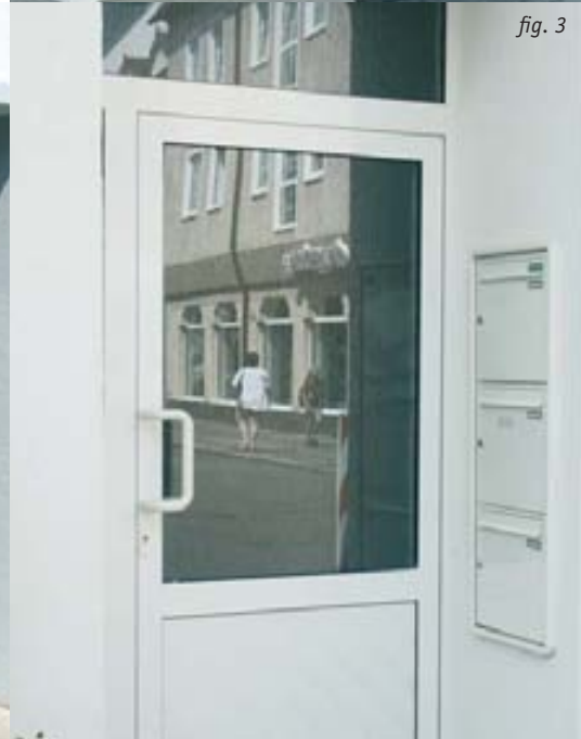
fig. 3: Recessed mounted multi-unit with vertical mailboxes and plaster cover frame TE 120
